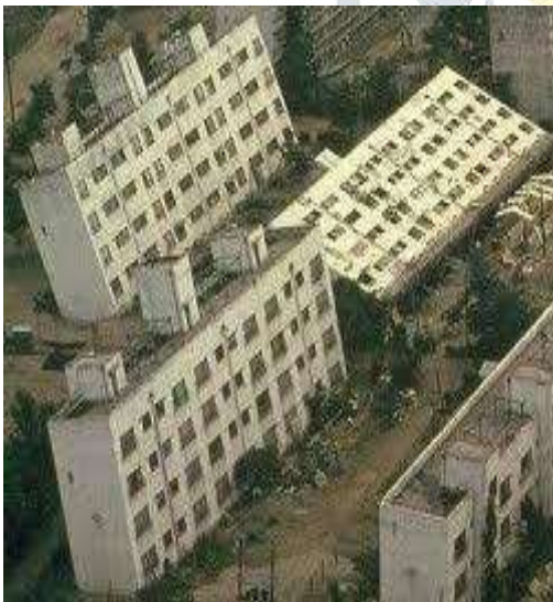
fig 1: tilting of apartment buildings at (courtesy of usgs)[1]
