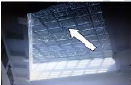
Light source enter the building through BIPV panel
