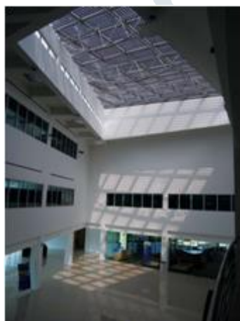
Atrium with glass semi-transparent PV modules (11.64kWp)
