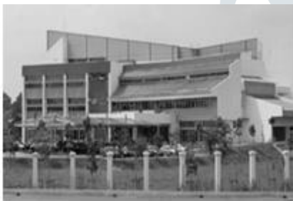
Building façade facing to the north
