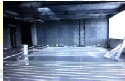
PEX pipe installed on the slab during the construction process.
