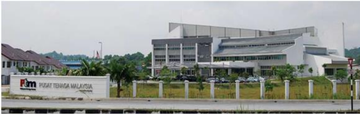
Colour of building exterior minimises heat gain
