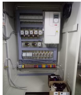
Figure 4 Wiring of VFD
