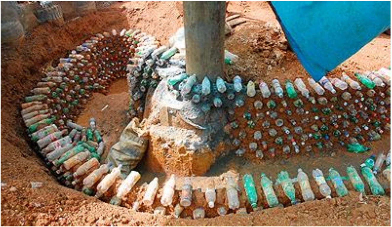
Figure 3.2: Construction of wall using Plastic Bottles (Earthship Karuna, 2007)
