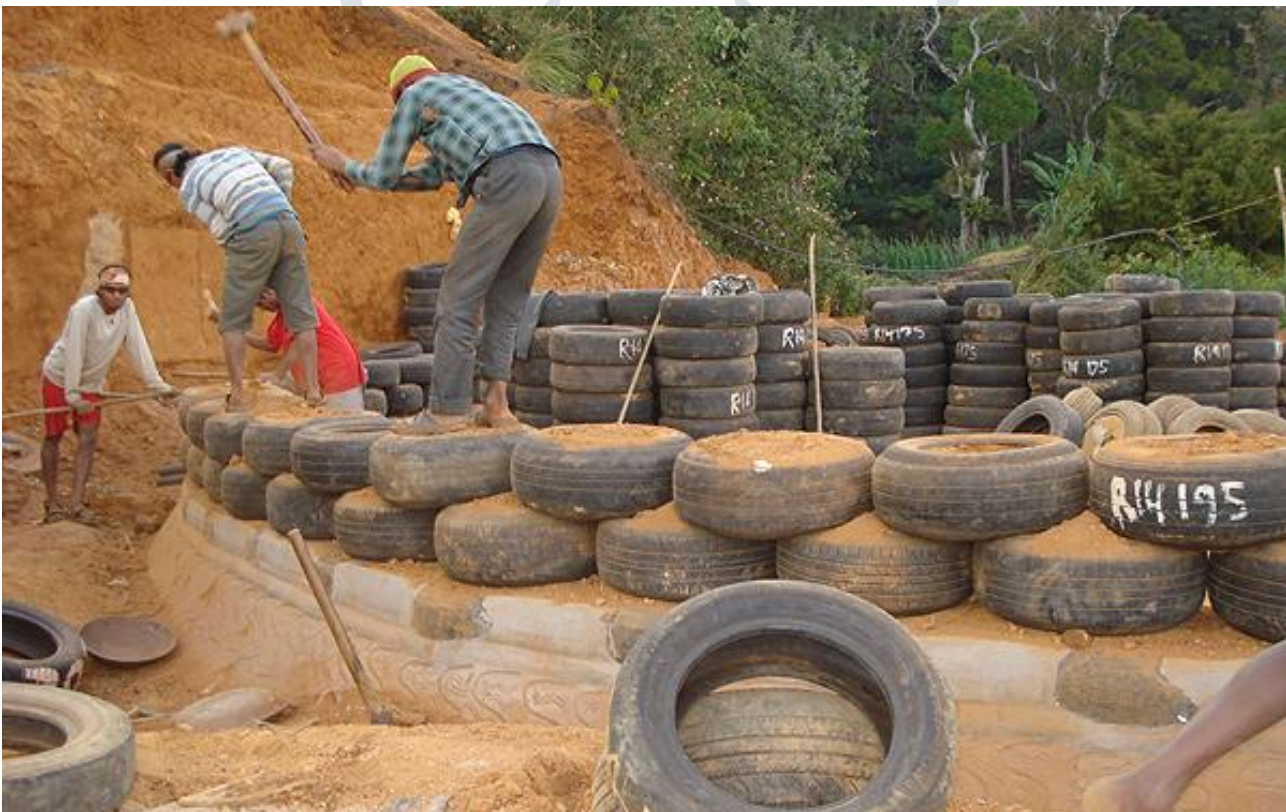
Figure 3.1: Construction using Rammed Earth Tyres (Earthship Karuna, 2007)
