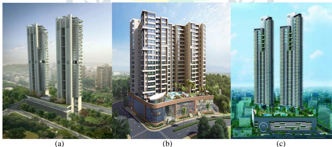
Fig-1: Podium Buildings (a) Oberoi Skyz-Mumbai (b) Bharat Sky Vistas-Mumbai (c) Orchid Heights-Mumbai.
