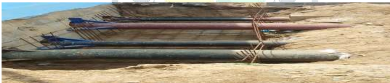
Fig:- Distributing water to GLBR'S
