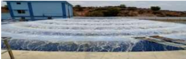
Fig:- Cascade areator
