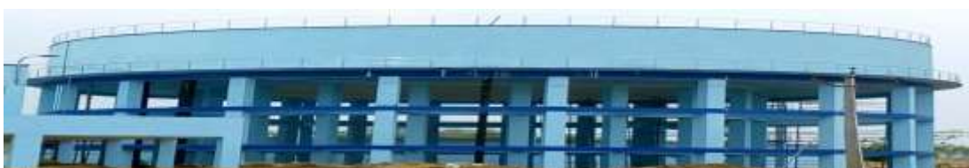
Fig:- Back wash tank
