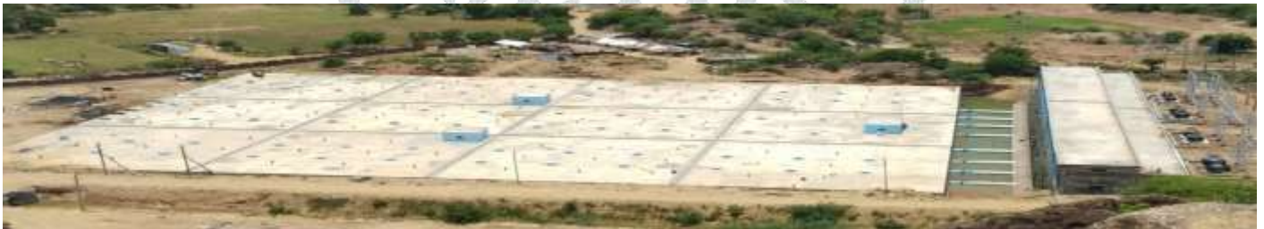
Fig:- 30000KL Clear water sump
