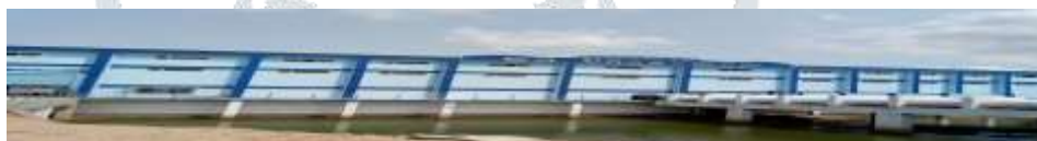
FIG:- Intake Constructed at Palair reservoir
