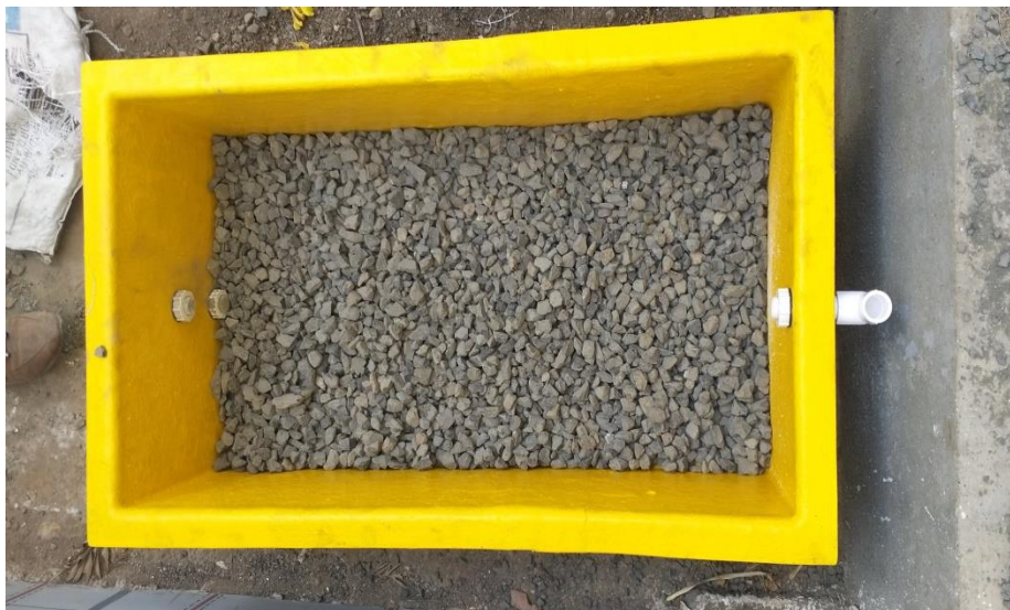
fig. no. 5.1.2 layer of aggregate
