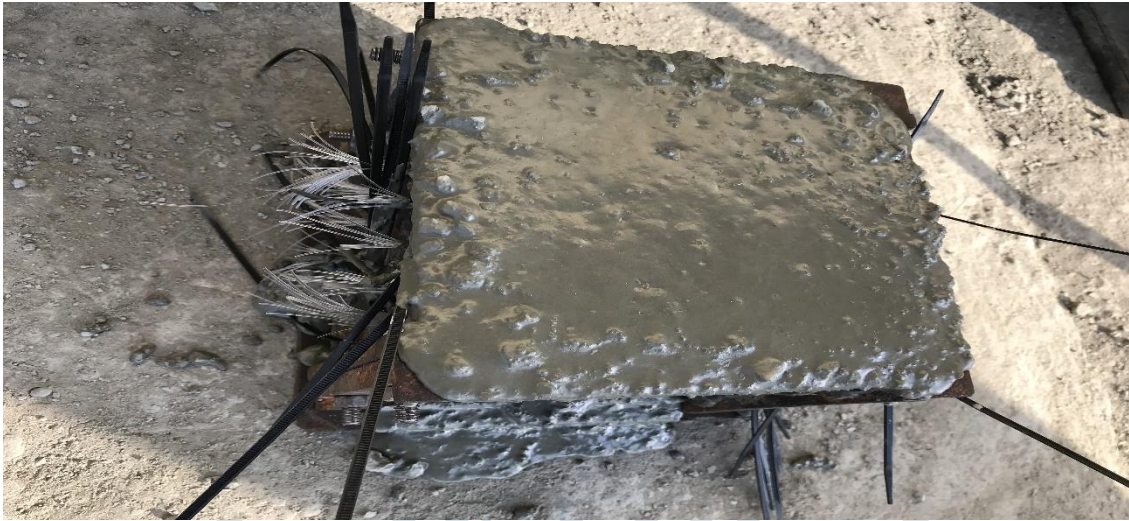
Figure :After Compacting Back
