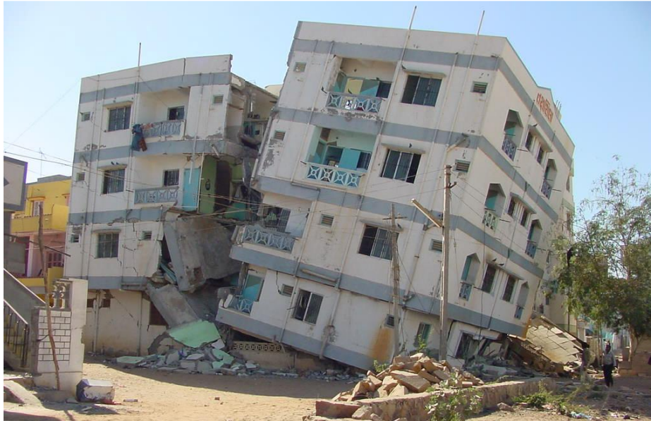
Figure: (c) RC Frame Buildings collapsed during 2001 Bhuj earthquake.
