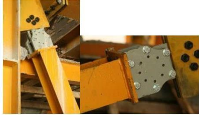
Figure 4: PVD Damper Installation
