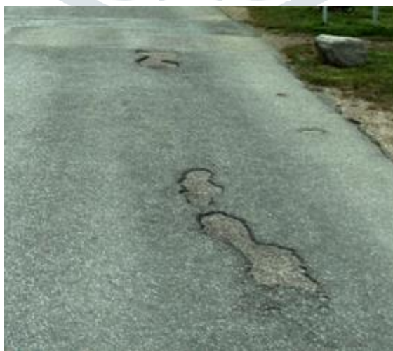
Figure 1. A pothole caused by fatigue failure
