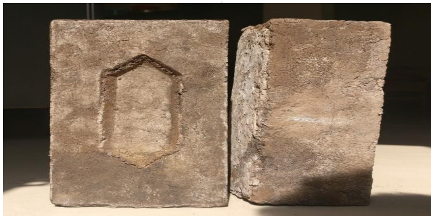
Figure 7: Modified brick sample showing the effect of efflorescence.
