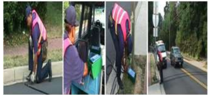
Fig 1: Installation of pneumatic tubes (photo credit: www.arlingtonva.us )
