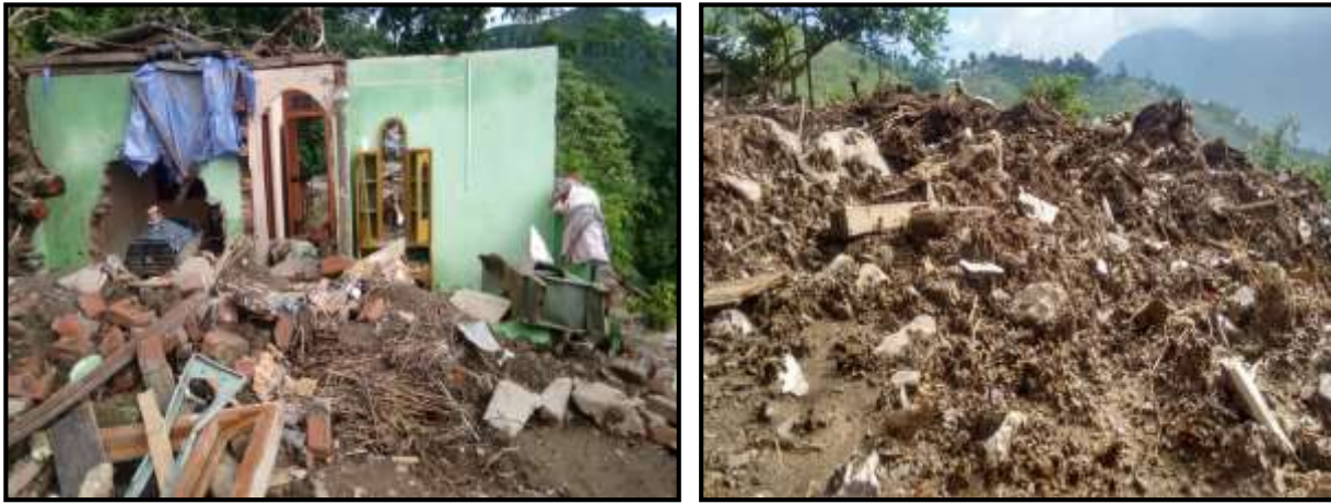
Plate 1: Destruction caused by the 2015 landslide in Limbugaon
