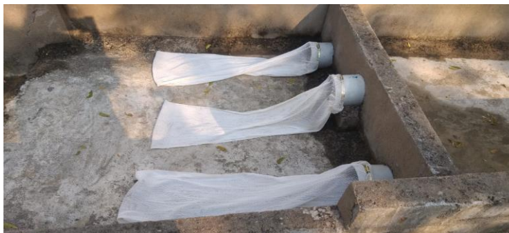
Fig. 4. Drainage Socks and Socks Passage
