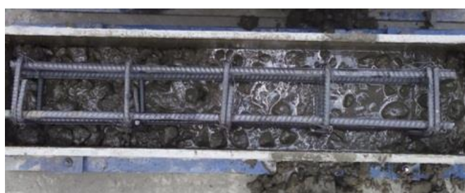
Fig.5 reinforcemnt placed in mould
