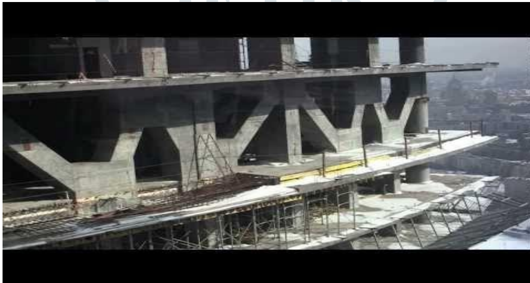
FIG 1.2. Concrete outrigger
