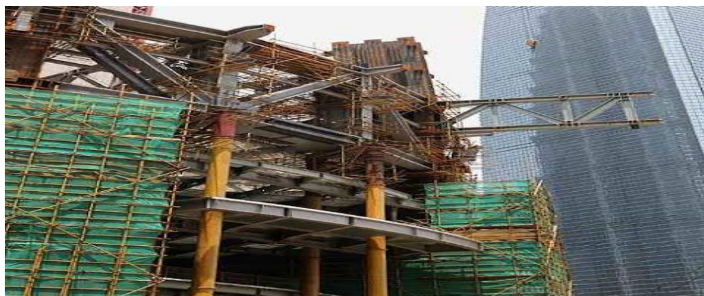
FIG 1.3 Steel outrigger
