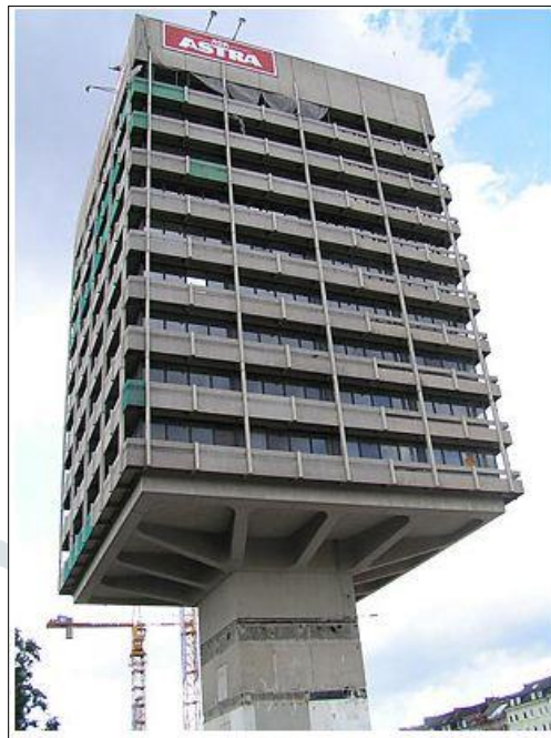
Fig.2.3 The Astra building in Hamburg, Germany
