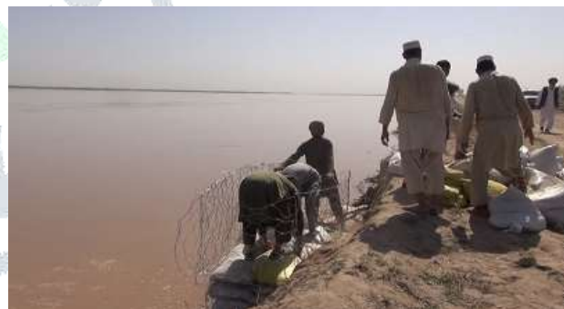
Fig2: Temporary embankments at Kunduz province – Pyanj Amu River
