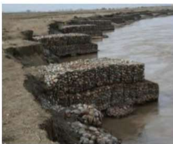
Fig. 11 Gabion embankment baskets to arrest bank erosion
