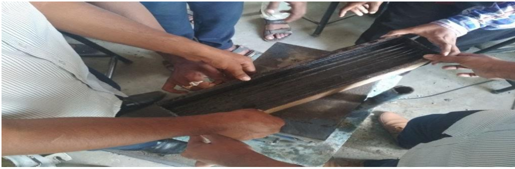
Fig. 7: Concreting the Mould
