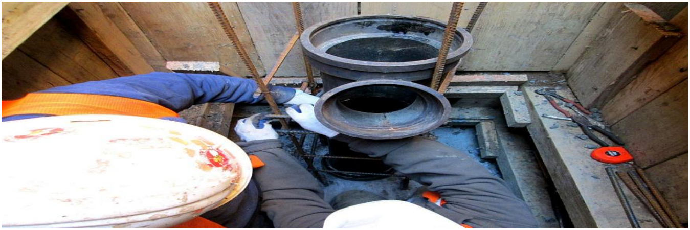
8" Riser Connection Being Built
