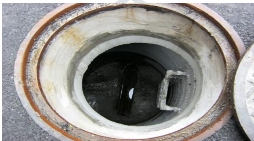
Finished manhole built by Balkan
