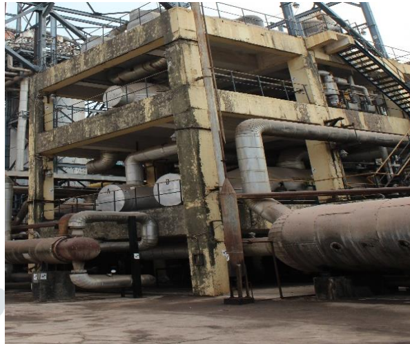
Picture 1 Real View of the building Table 1 Building data
