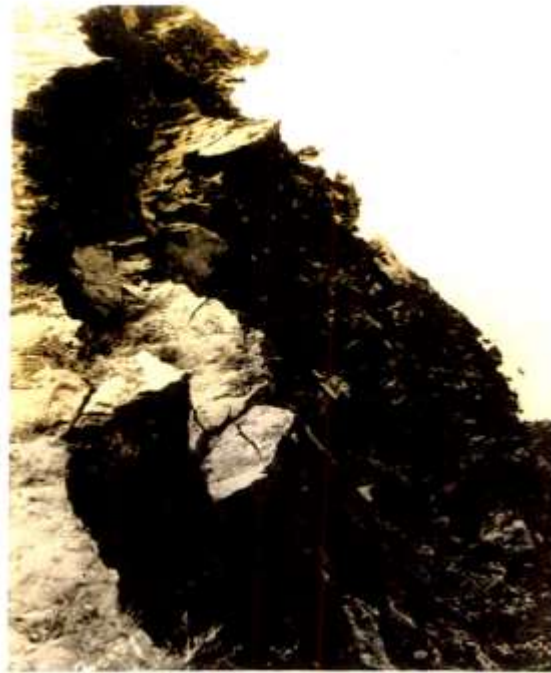
Figure 1.3: Increase of the erosion process due to the circulating water, the bank of the river gradually recedes at Patuli.
