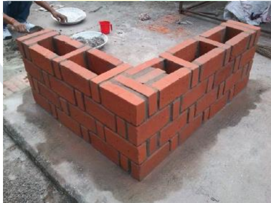
Figure1. Rat trap bond mechanism
