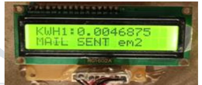
Fig. 8 LCD display showing Energy Meter 1 Readings
