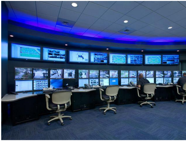
Fig 3 View of Smart Cabin
