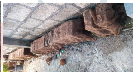
Fig 2.2 Curing of brick triplets Fig 2.3 Covering of brick triplet with gunny bag
