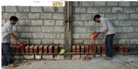
Fig 2.2 Curing of brick triplets Fig 2.3 Covering of brick triplet with gunny bag
