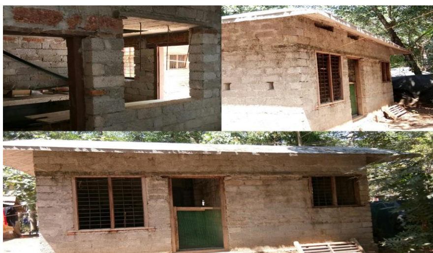
Fig 3.1 Present situation of PMAY and LIFE MISSION homes
