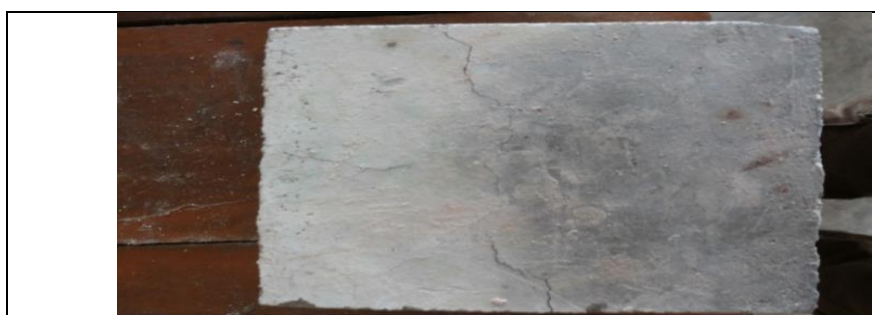
Figure 6 : Copper slag Concrete after exposed to 600° C
