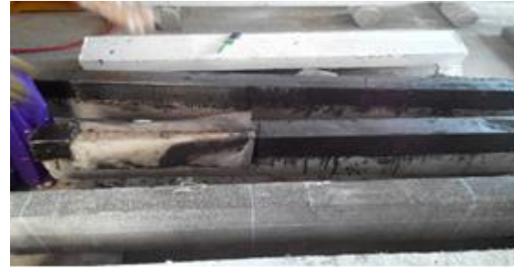
Fig 5: Wrapping Of Double Layer Of Carbon Fiber Mat
