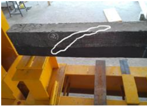
Fig 12 crack pattern on CF-2L Beam
