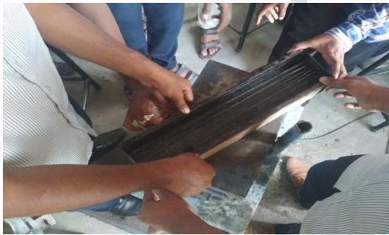
Fig 4: Concreting the Mould
