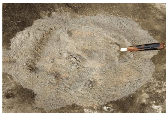
Figure 3. Mixing of ECC concrete.
