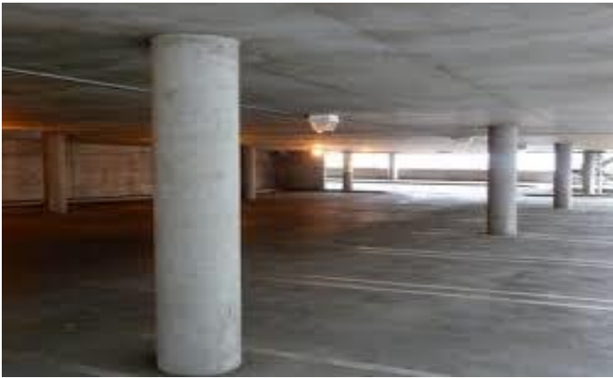
Fig. 3 : Flat Slab without Drop
