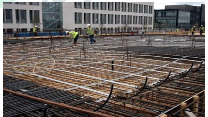
Fig. 8: Reinforcement in Flat Slab
