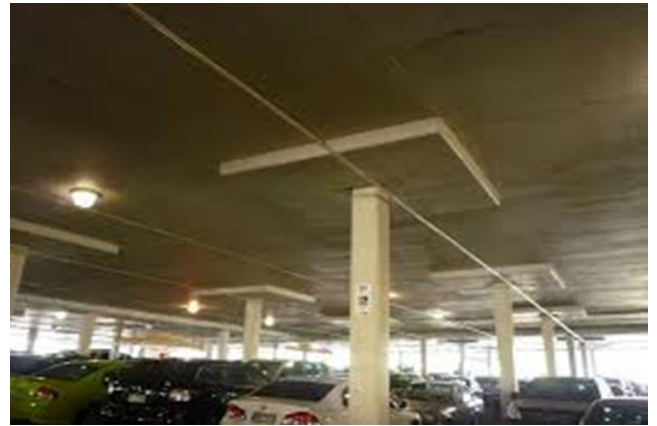
Fig. 4: Flat Slab with Drop
