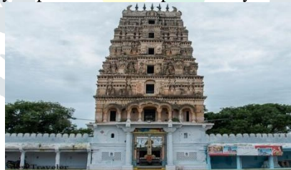
Fig 1 Front face of the historical structure
