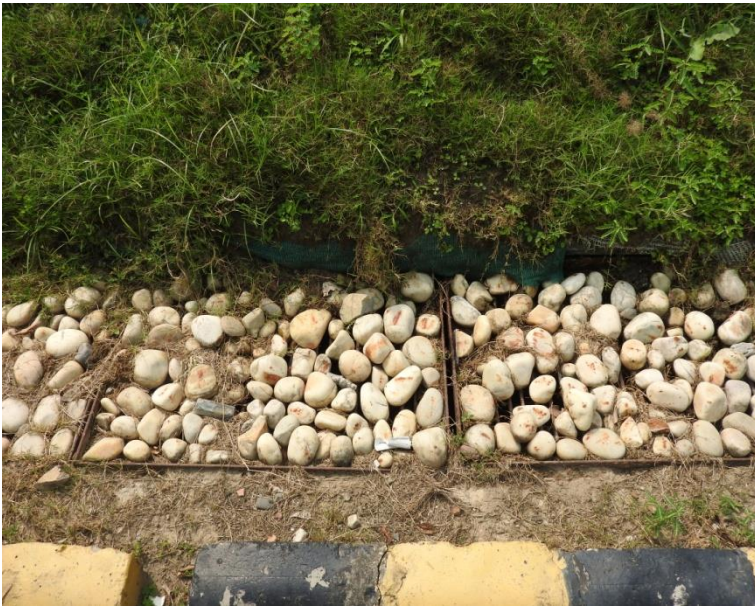
Drains taking water to Rain water harvesting through gravity Source: Researcher
