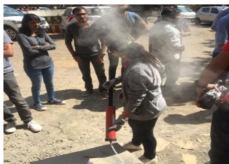
Fig.5. Cleaning of holes (Blowing)
