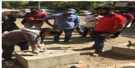
Fig: 8. Inserting HIT-V rods
