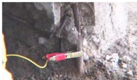
One end of Half-Cell connected to the reinforcement
