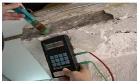
Half-Cell Potential Test of Slab
