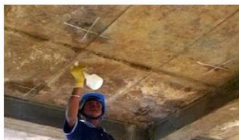
Marking of Slab and Pre-wetting for Half-Cell Potential Test
