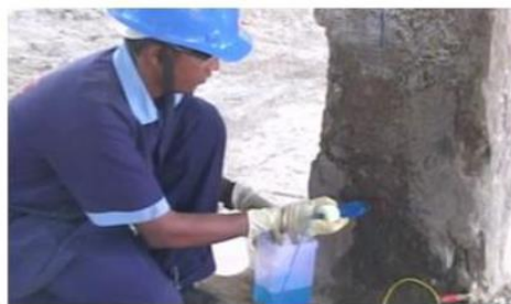
Half-Cell Potential Test of Column
