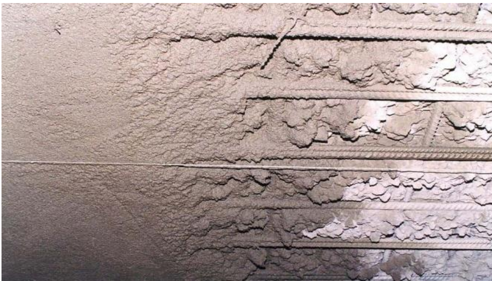
Fig.2 Concreting Of Fire Damaged Slab
