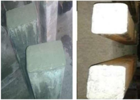
Fig No.3 CFST Column BeFor After Application of Curing Compound
