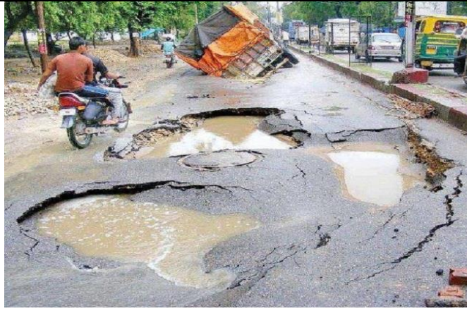
Fig 1.2 Road Conditions in Kerela
