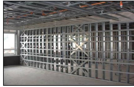
Figure 2 LGS framing before the sheeting has been done (Source: www.understandconstruction.com )
