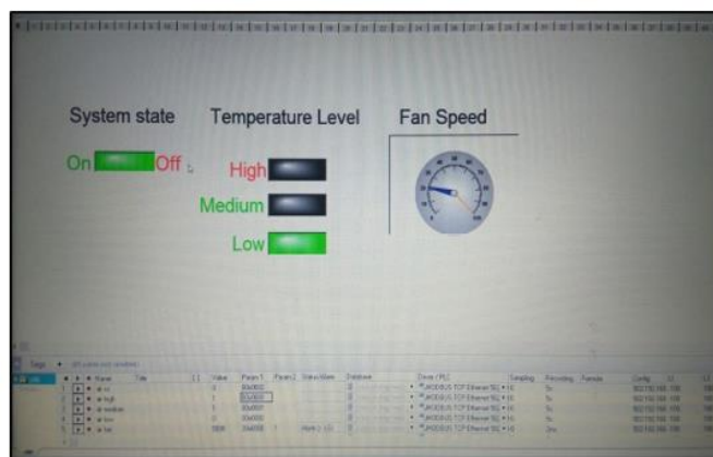
Fig 7 SCADA Setup Conditions-1
