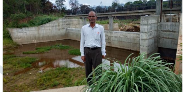
d) U/S of weir constructed inside the Kadumane estate across Kadumane estate Halla - 1
