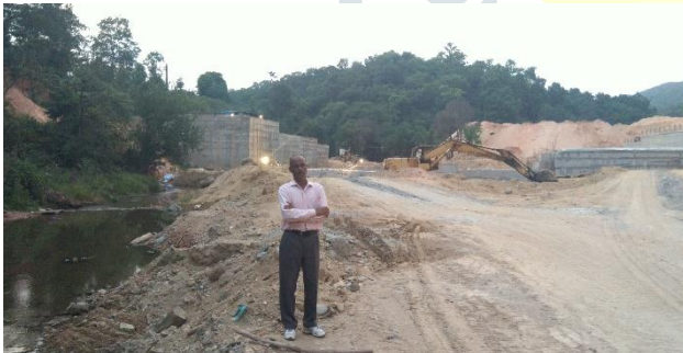
g) U/S of weir under construction near Kadaravalli across Hongadahalla Halla
