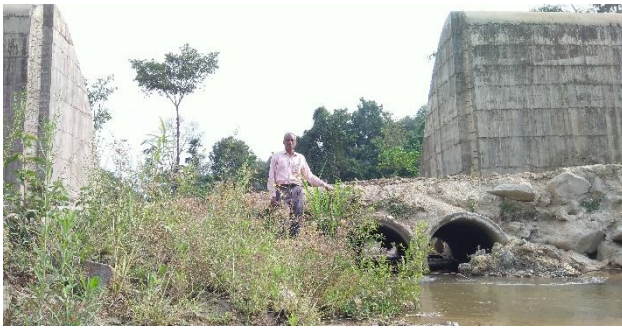
a) U/S of weir under construction near Kumbaradi across Yettinahole
