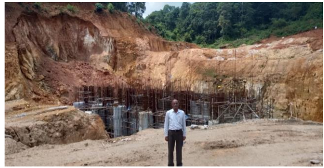
b) Pumping house under construction in Kadumane village across Kadumane Halla
