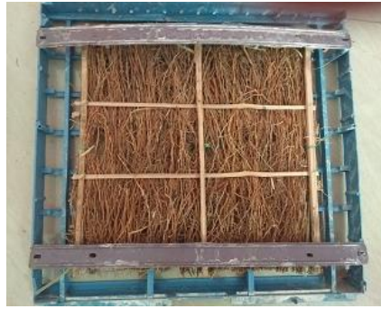
Fig.no.9. Installation of Khus pad
