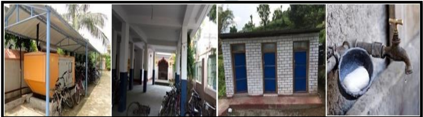
(Generator facility, cycle stand, toilet rooms, drinking water facility)
