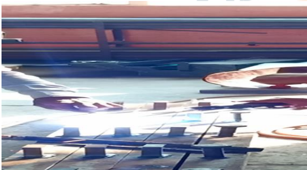
Fig.4 Cttng and welding process on profiled deck sheet
