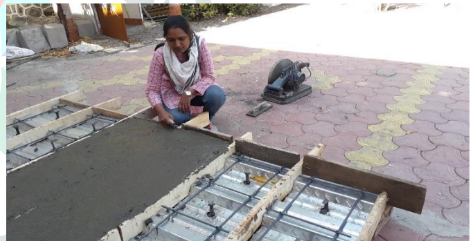
Fig.5 Concreting process on composite slab
