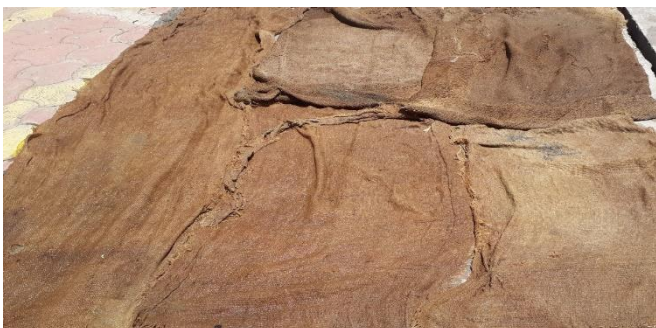
Fig.6 Curing process on composite slab
