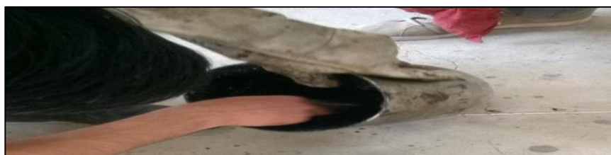
Fig 4: Mixing of bituminous concrete
