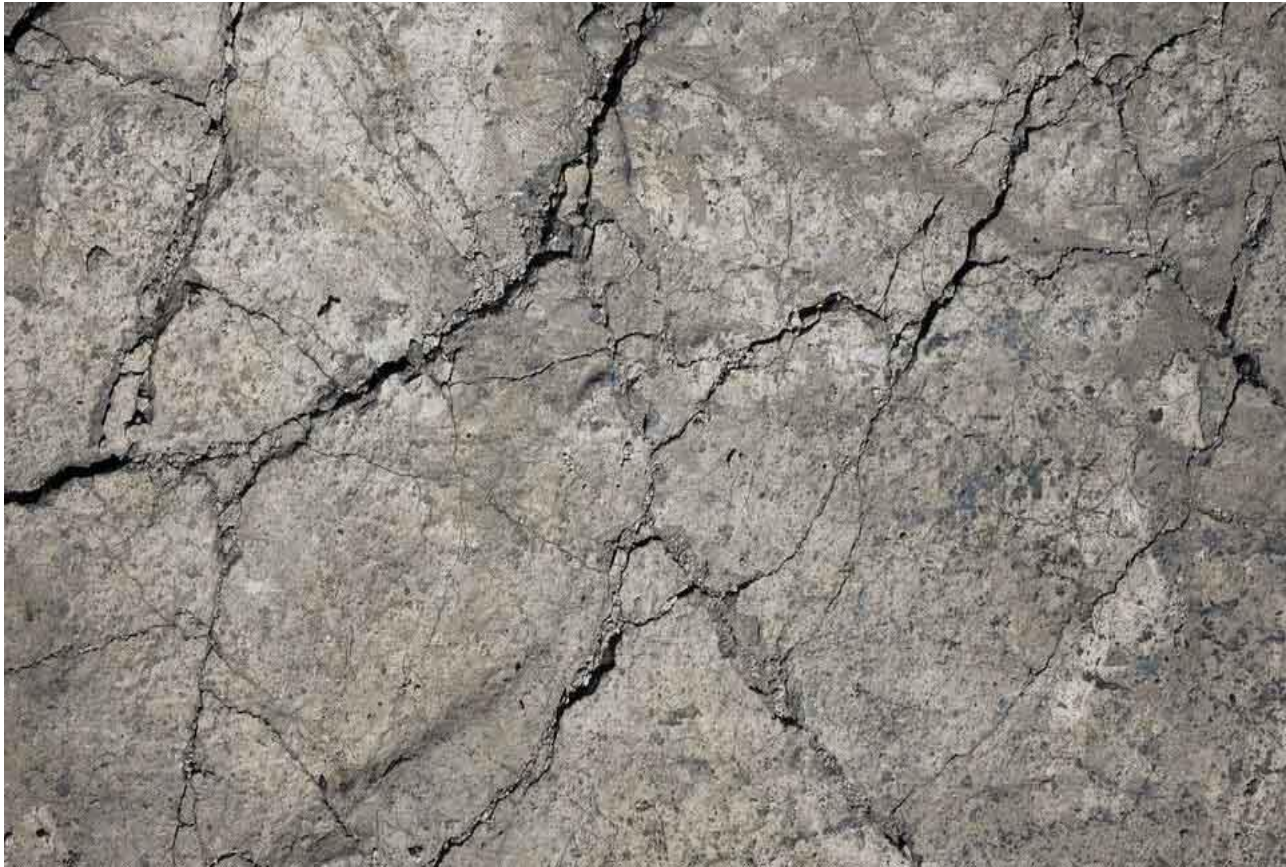
Figure 1.1: Cracked concrete
