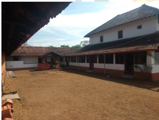
Figure – 2 View from courtyard
