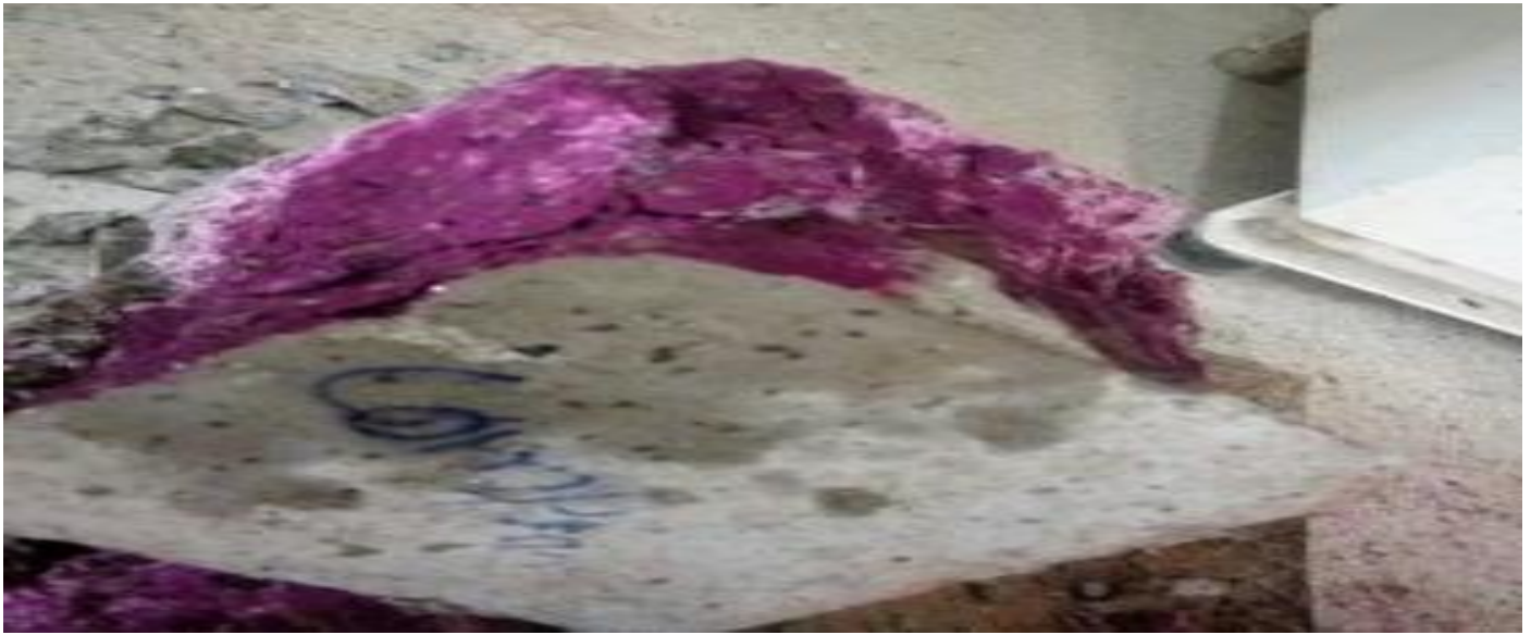
Fig.7: Carbonated Concrete Sample
